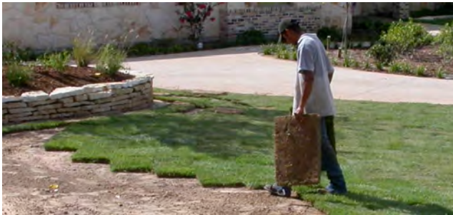
Figure 4. Sod installation
